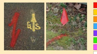
Electric power lines Gas, oil or steam pipelines Communications lines, cables or conduit Potable water Reclaimed water, irrigation and slurry lines Sewers and drain lines Temporary survey markings Proposed excavation
